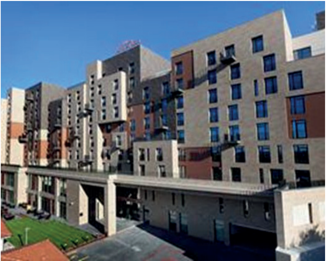
Hilton İstanbul Beyoğlu Sütlüce project of FERMAK Inc., which is among the companies VEO is cooperating with on projects basis
