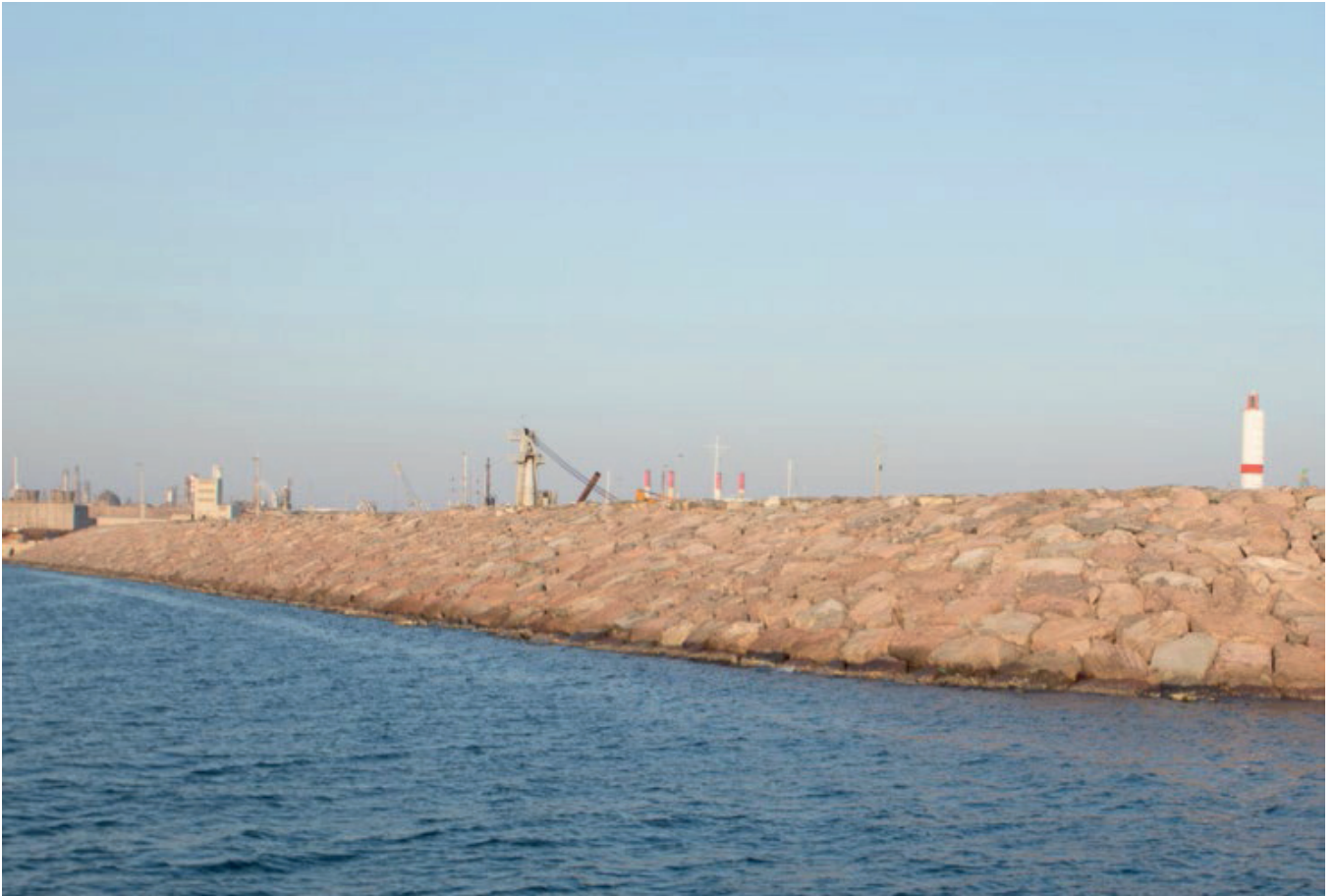
Views from Petkim Container Port project of FERMAK Inc., which is among the companies VEO is cooperating with on projects basis
